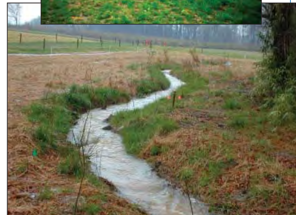
Figure 5.7 Yates Mill Pond tributary-restoration project after construction
