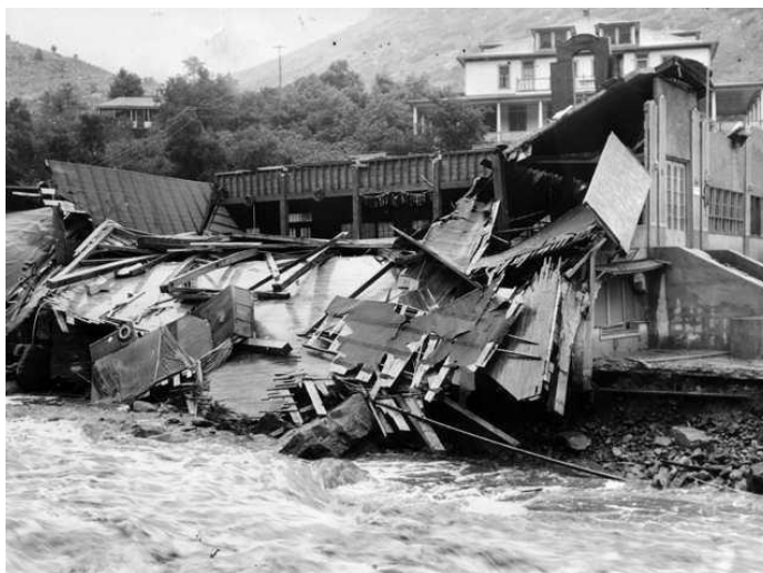
Figure 3.52: Photograph of Eldorado Springs Resort's destroyed dance pavilion after the 1938 flood. "Eldorado Springs Flood, 1938," Denver Public Library, https://history.denverlibrary.org/gallery/pool-party-eldorado-canyon#PhotoSwipe1598896032534 .
