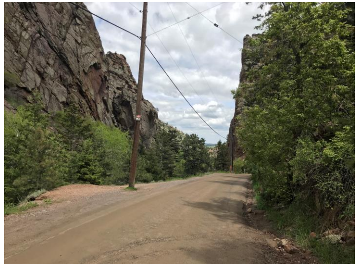
Figure 4.6. The main Park road that travels along South Boulder Creek is narrow and easily becomes congested on summer weekends.
