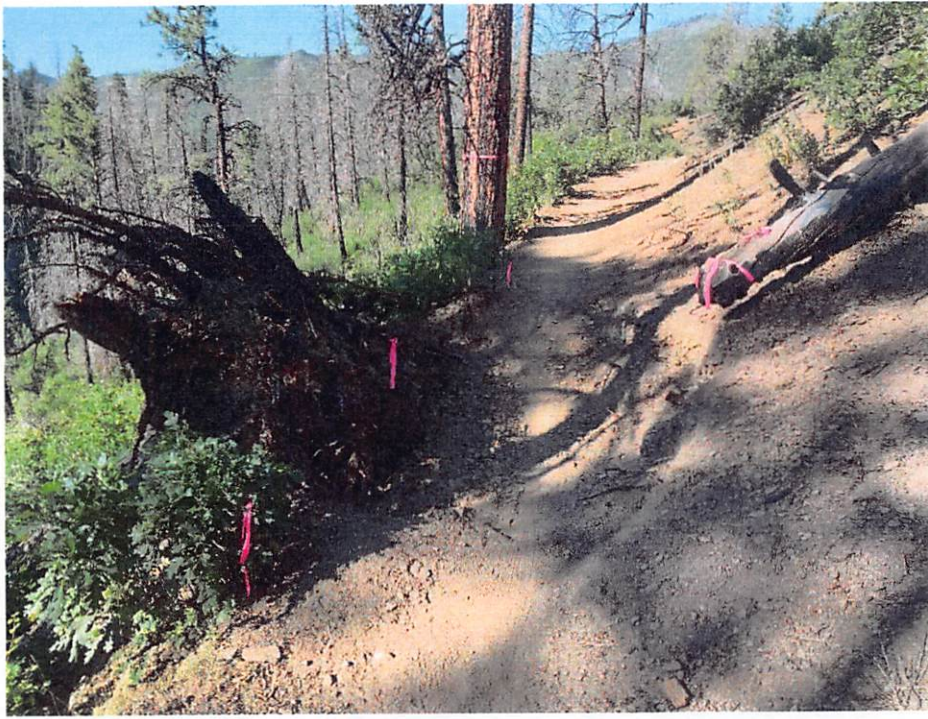
A Large crater formed on the Hermosa Creek trail when a ponderosa fell – the crew ultimately filled this in, but spring of 2024 will bring another visit to add more soil as it has compacted so much.
