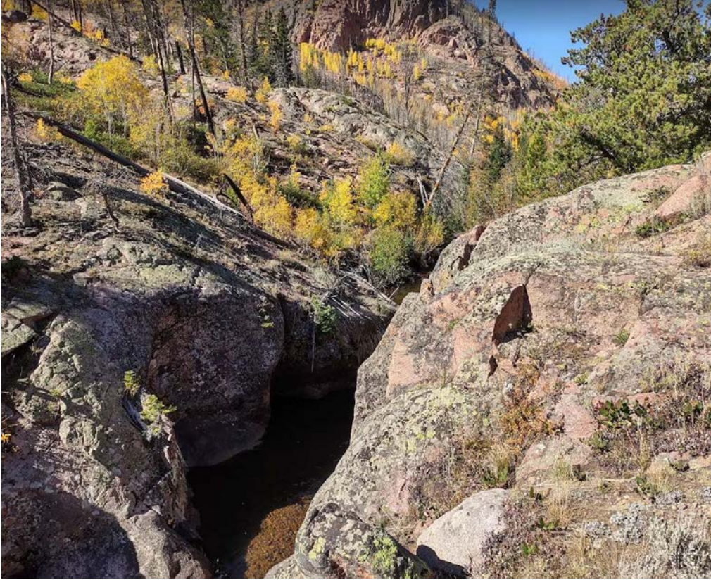
Figure 8 Proposed location of Red Canyon Bridge above slot canyon, just downstream of current crossing
