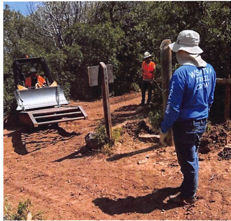
In Progress WSATVA Work Crew
