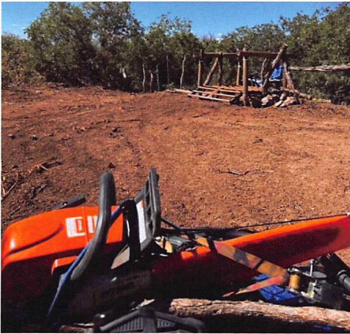
Work Done by Subcontractor
