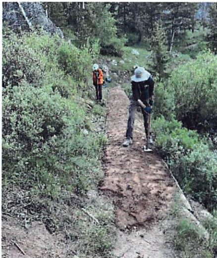
RMYC Crew working to re-crown a turnpike on Wide Open (#9508)
