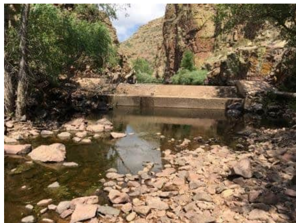
Figure 5-2. Calloway Diversion Structure
