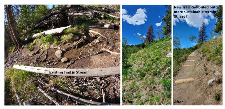
The lower trail re-routes will preserve the wet areas that are currently seeing excess amount of soil erosion during the spring melt and large rain events. The continued construction of the lower re-routes will relocate the trail to more a more sustainable location that will drain more effectively and preserve existing riparian habitats.
