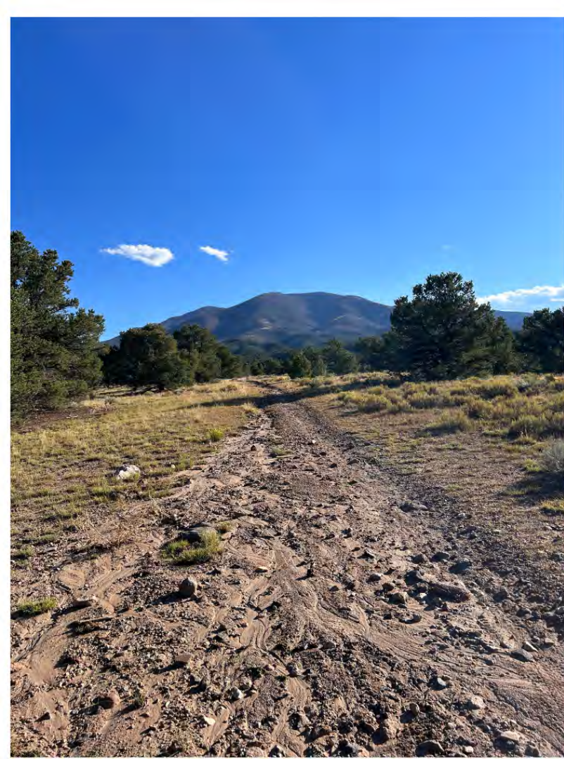
Img. 1 – Washout on Race Track (August 2023)
