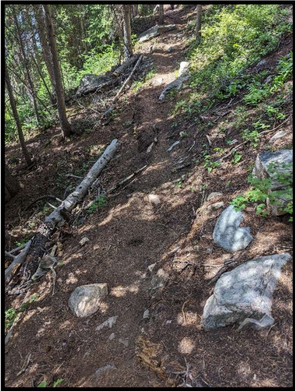
(South Park RD - Jefferson Lake Loop Trail, eroding sections of tread requiring new retaining walls and reconstruction)
