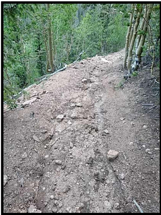
(Pikes Peak Ranger District – Elk Park Trail, washed out trail sections requiring corrected waterbars and assessment for potential new alignment)
