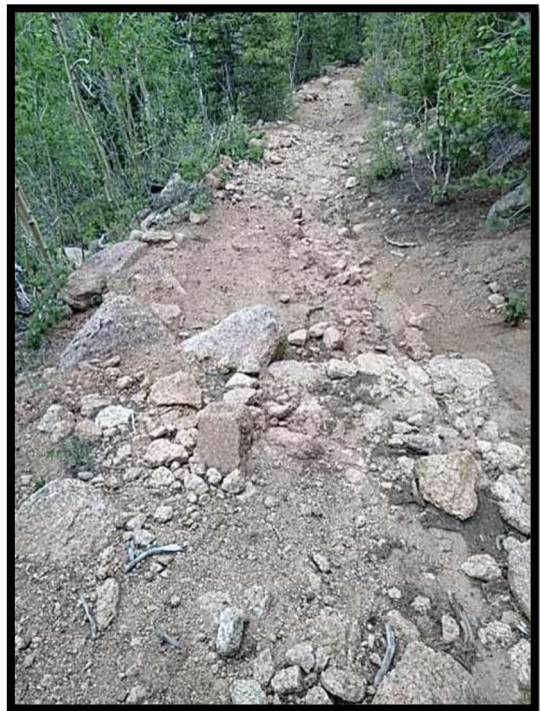
(Pikes Peak Ranger District – Elk Park Trail, washed out trail sections requiring corrected waterbars and assessment for potential new alignment)
