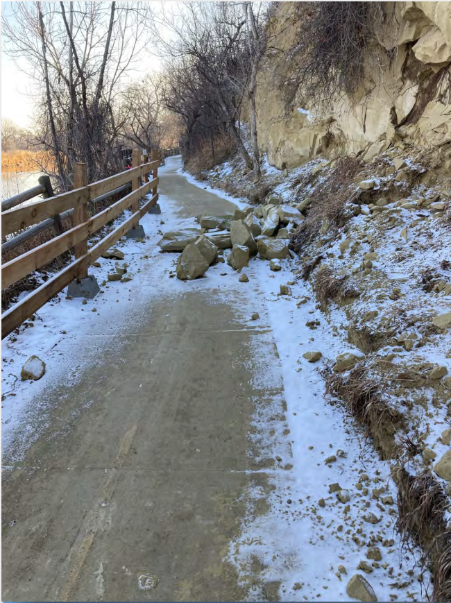
LEFT: Rockfall onto trail. This occurred shortly after the bluff face was scaled to remove loose rock. Face is inspected regularly for loose rock. (2021)
