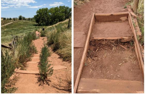
Devil's Backbone Open Space has 17 miles of trail. High use and torrential rains have caused damage to the trails system in 2023. Replacement of steps is needed on the high use Wild Loop trail (see photos of steps).
