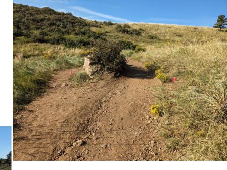
Horsetooth Mountain Open Space has 30.5 miles of trail. High use trails like Horsetooth Rock and Horsetooth Falls are always in need of maintenance to keep water off and users on trail. Both photos show damage to the Horsetooth Falls trail due to higher-than-normal moisture received in 2023. On this section of Horsetooth Falls trail, 900 ft of trail needs rebenched with improved drainage to reduce muddy conditions and keep users on trail.
