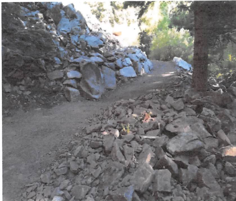
trail section reconstructed for safe passage
