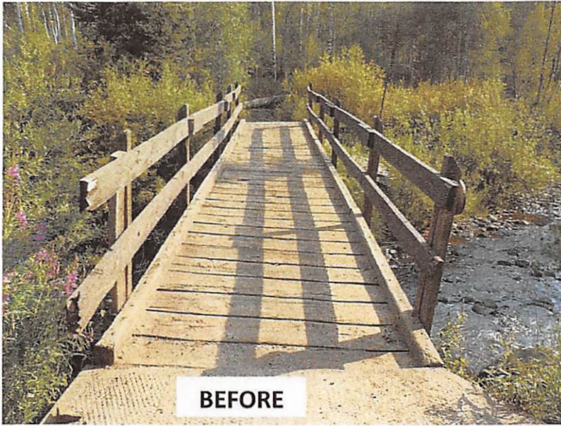
Surface Creek Bridge Deck and Railing Replacement
