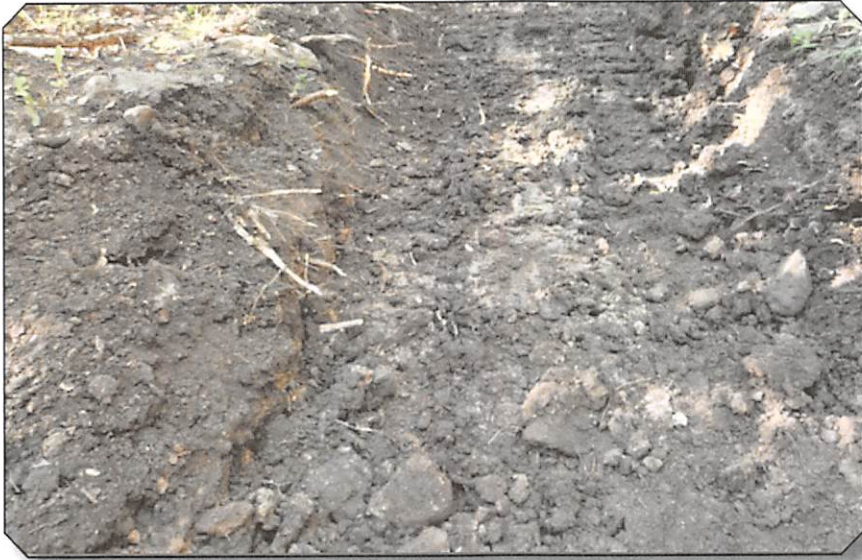
AFTER PICS OF SEVERE MUDHOLE AND PROCESS INVOLVED
