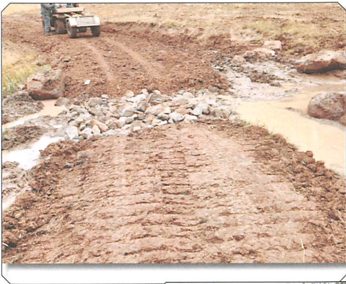
PICS THAT SHOW WATER PROJECT, WHAT TO DO TO GET A MUDHOLE PROPERLY DRAINING AWAY FROM TRAIL
