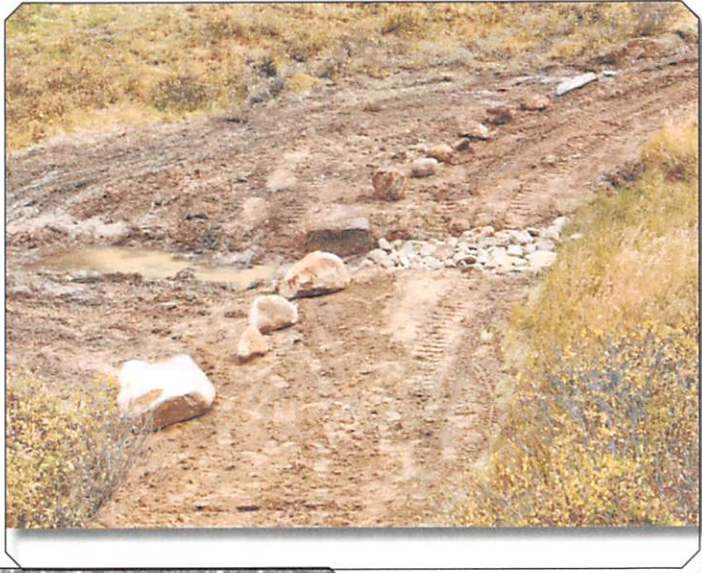
PICS THAT SHOW WATER PROJECT, WHAT TO DO TO GET A MUDHOLE PROPERLY DRAINING AWAY FROM TRAIL
