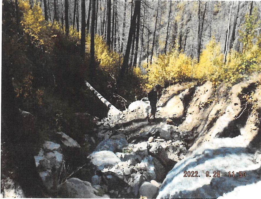
Hermosa Creek Trail looking down trail from inside washout
