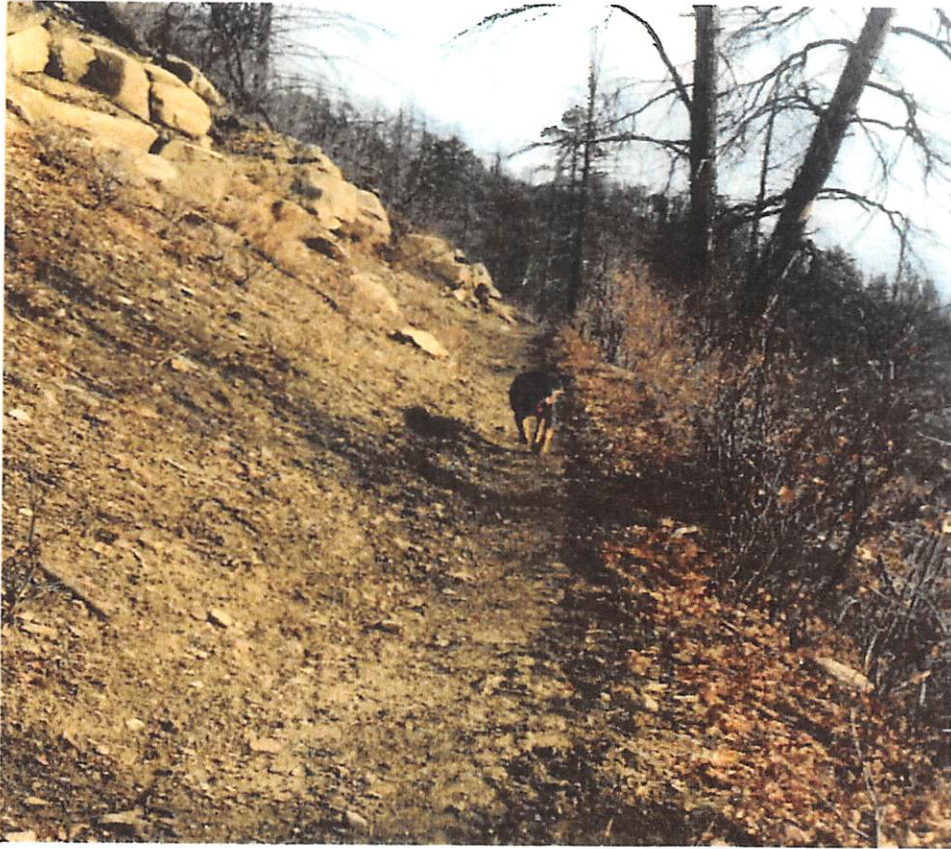
The scope of work for the SCC project included benching to widen the trail and re-establish sustainable, functional tread.
