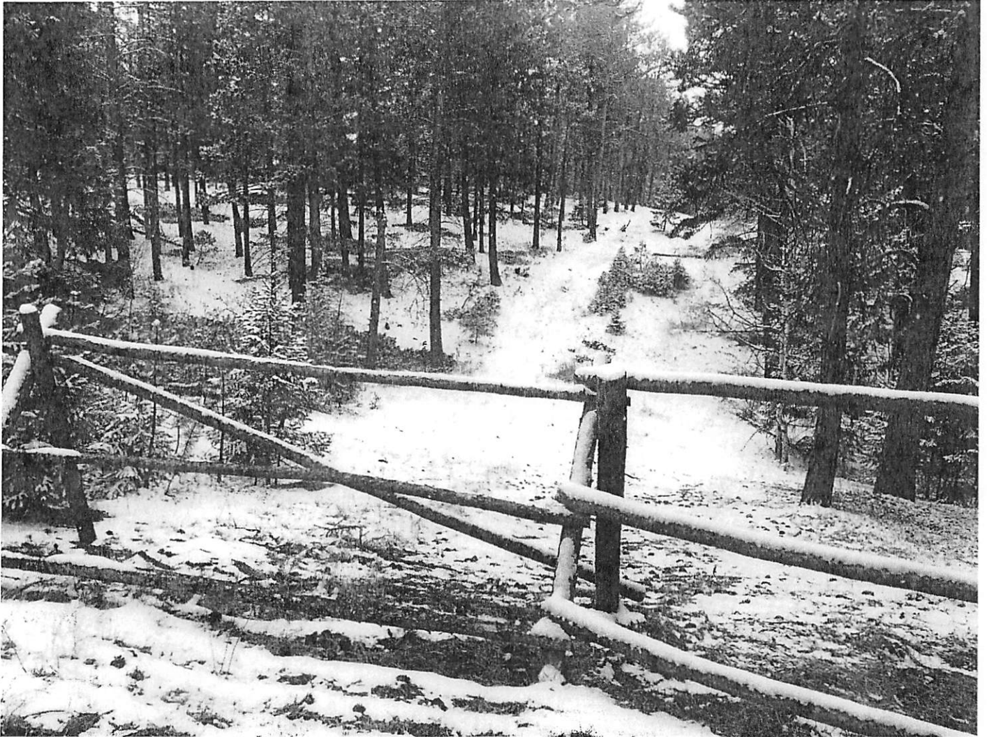
Fence construction to protect rehab areas
