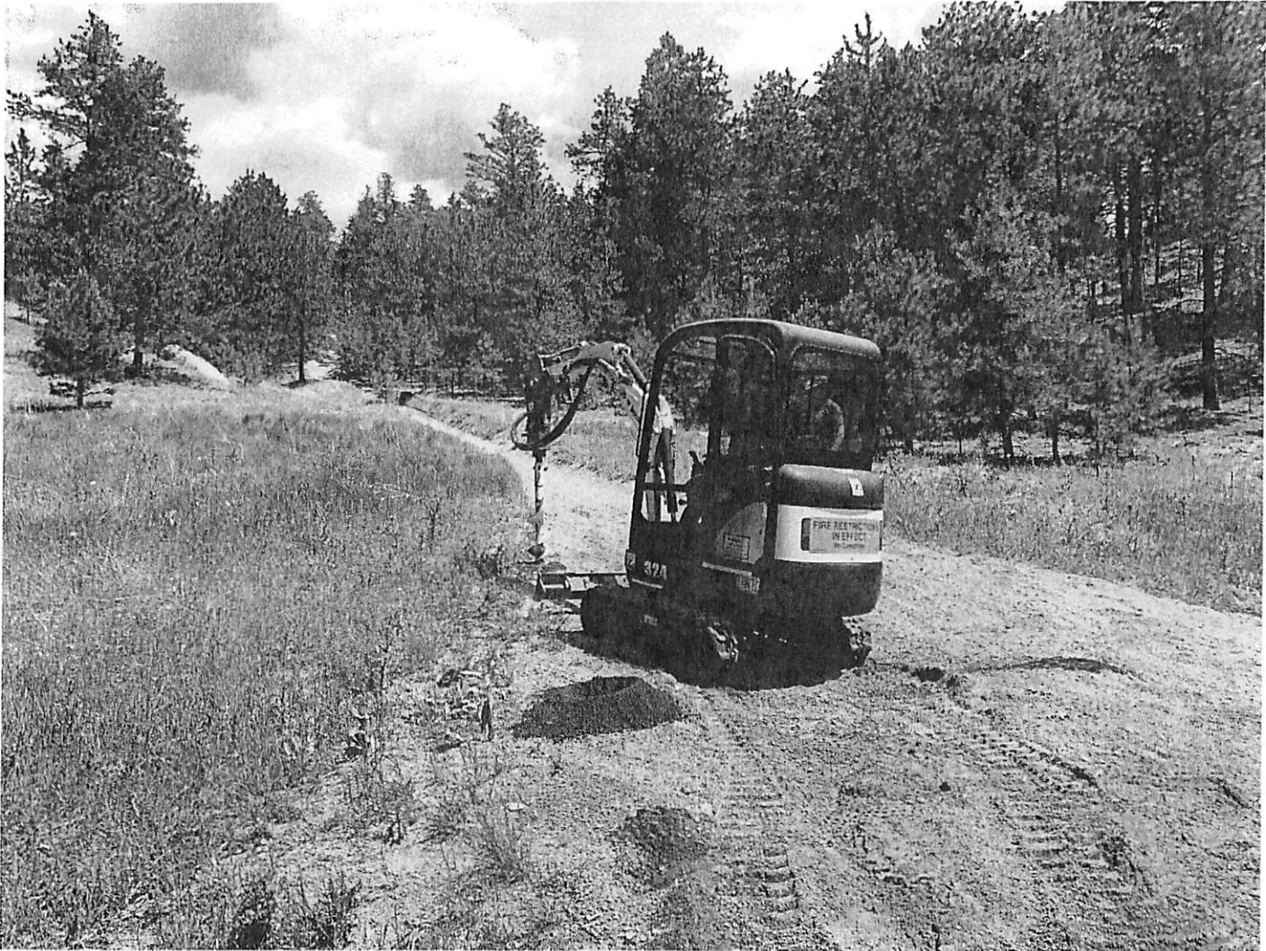
Post and cable install to minimize trail width
