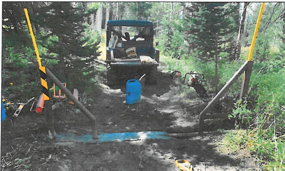
Typical width restrictor gate installation on a 62" or less UTV trail.
