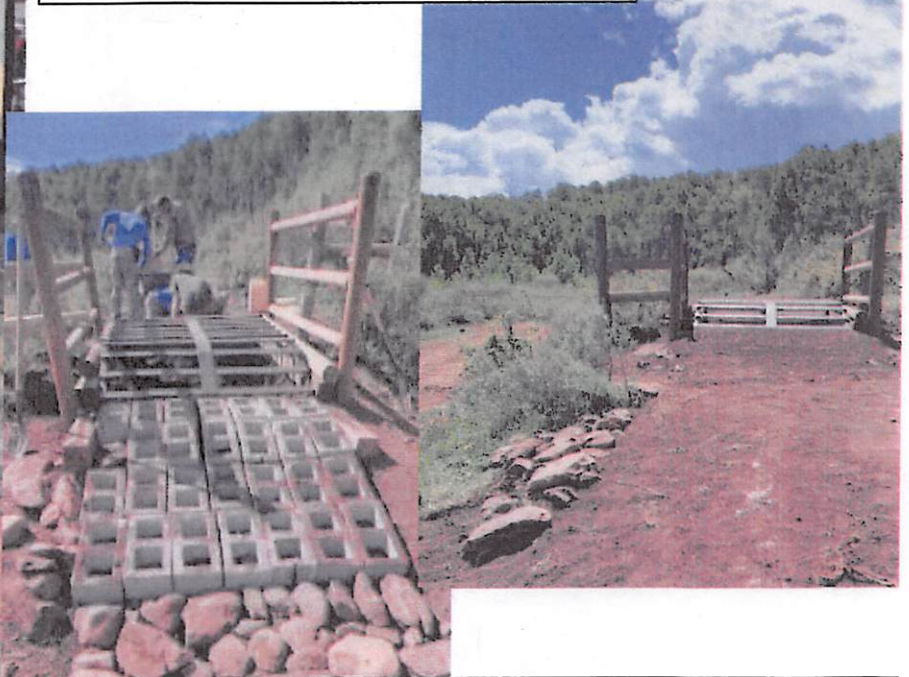
Cattleguard install with WSATVA on Powerline Trail #520 located on the Grand Mesa
