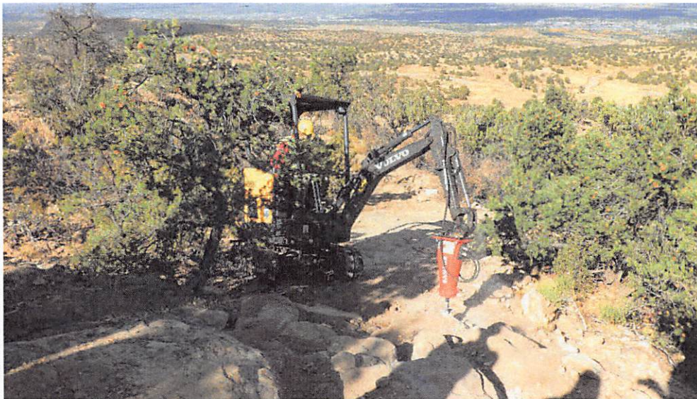
Using rock breaker to improve Quad Rocker trail tread and possibility.
