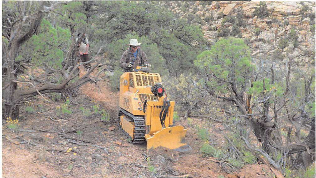
Operating new trail dozer on Cedar Point.
