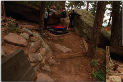
Above: The Pebble Boulder hosts a number of classic bouldering problems and was identified with Flatirons Climbing Council (FCC) as having suffered significant erosion around the base of the boulder. Over the years, feet of soil loss have exposed tree roots and rocks making for a difficult landing. All runoff coming downhill wraps around the boulder from either direction creating a significant trough. In the photo above, the first step and tier of wall has already been installed.
