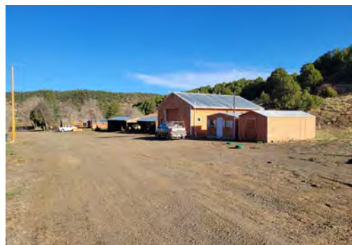
Exit 8 Maintenance Shop and Outbuildings
