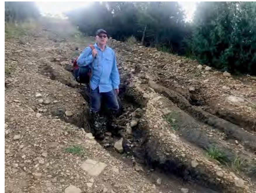
Flood Damage on Ranch Roads Creating Gullies 3-4' Deep
