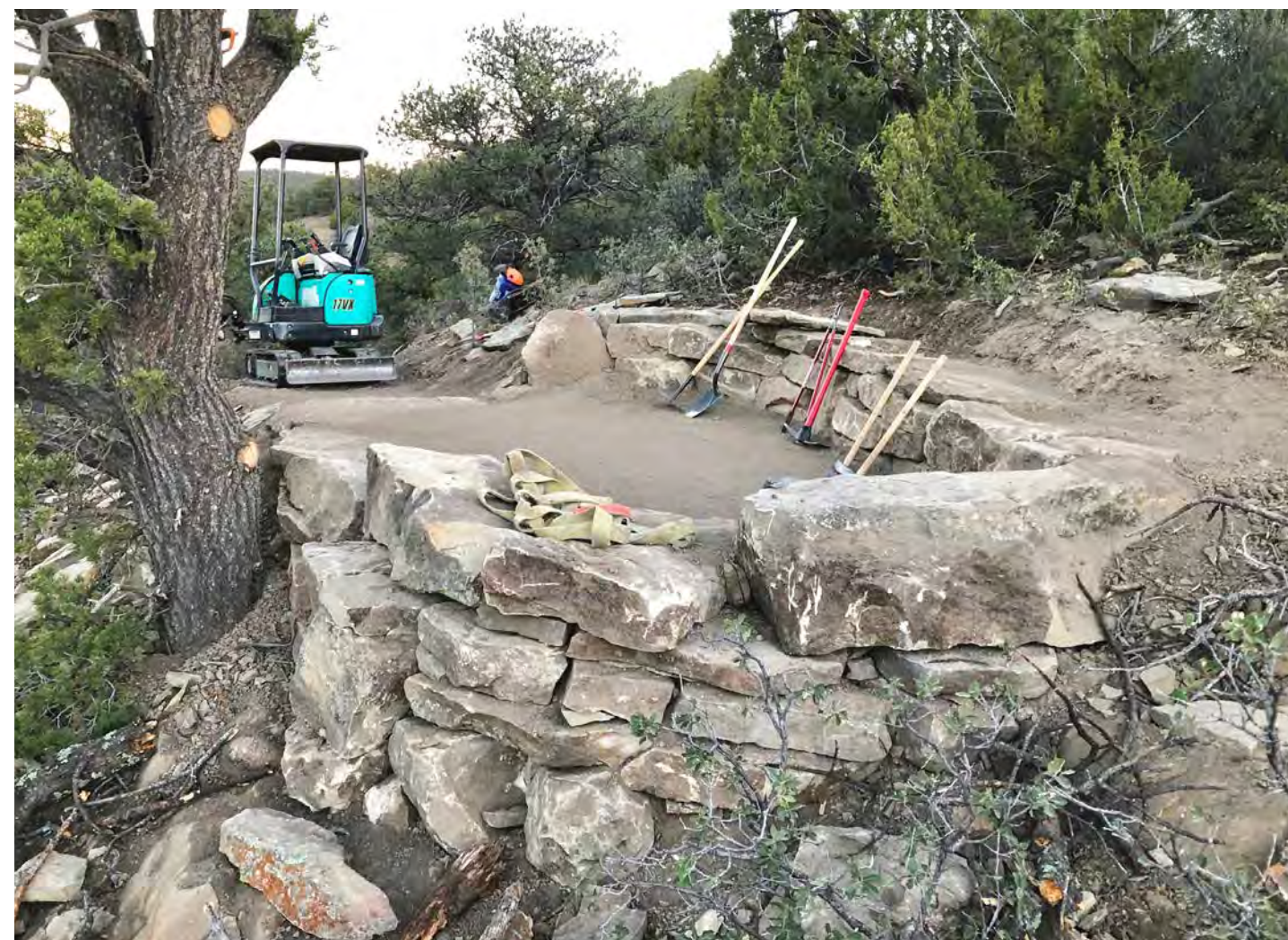
First Look Trail Construction
