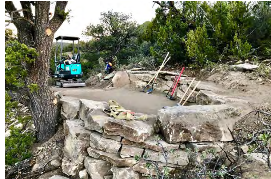
Showing Dry-laid Stone Retaining Wall on the First Look Trail
