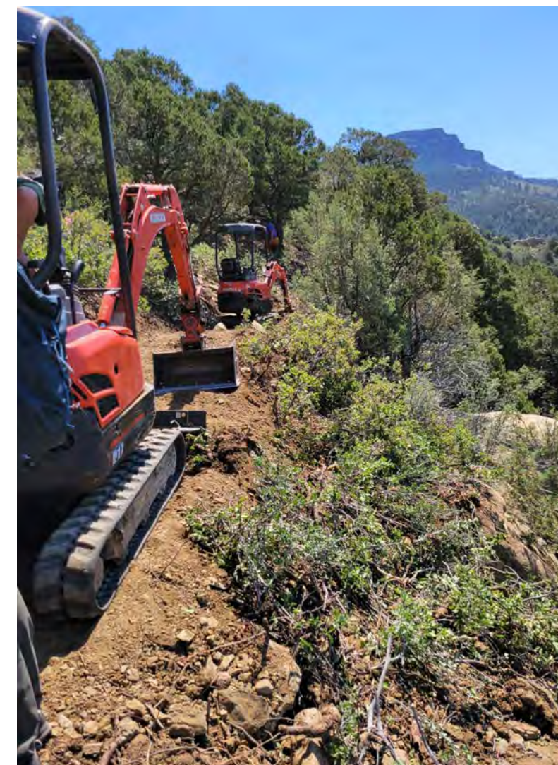
Construction of the Fishers Peak Trail
