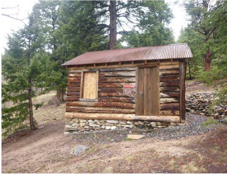
Photo 30. Bootlegger’s Cabin after stabilization work, May 2015.
