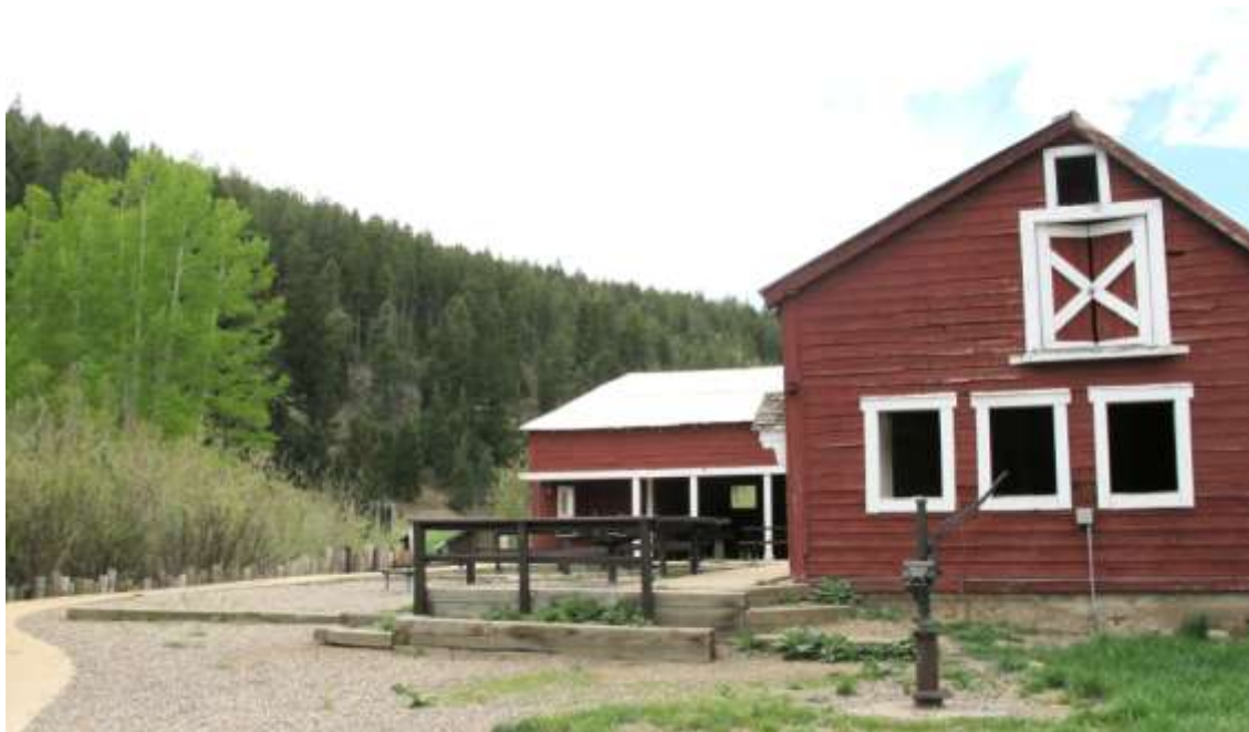
Main Entrance & water pump
