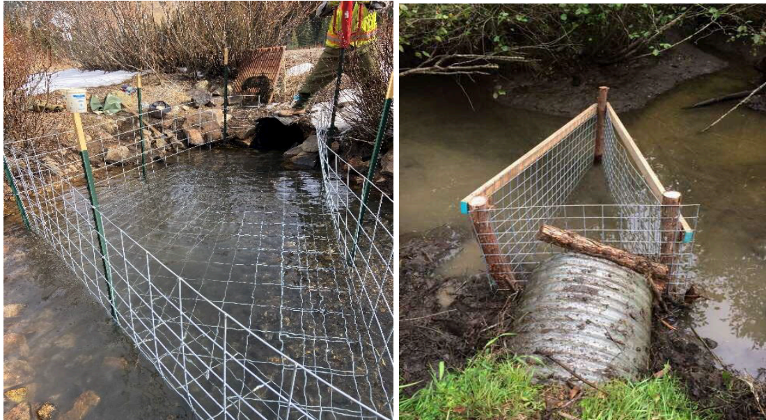
Left: Photo by Rory Cowie, Alpine Water Resources, LLC, Silverton, CO, showing a classic triangle keystone design. Right: Photo from Best Management Practices for Resolving Human-Beaver Conflicts in Vermont (2017) showing a smaller triangle design to fit the smaller space available.
