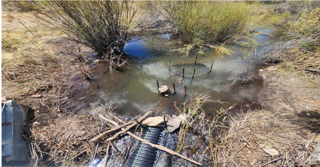
Photo provided by the RGNF taken from upon the bridge looking down at the flow device built into a notch of the beaver dam.
