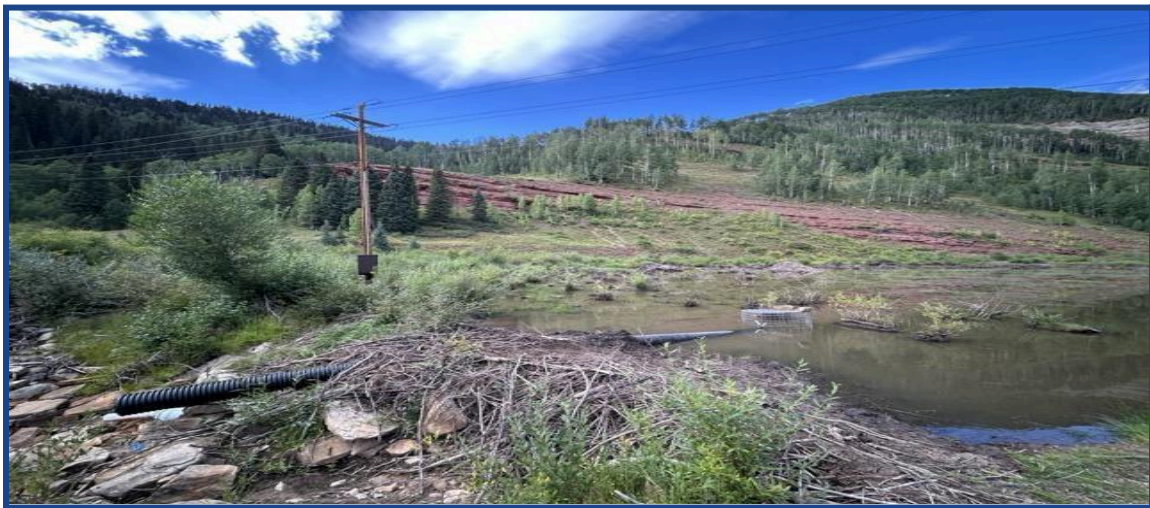
Photos #xx & xx from Rory Cowie, Alpine Water Resources, LLC, Silverton, CO, showing a classic example of when a pond leveler is needed to reduce the water level of a beaver pond located next to Hwy 145 near Rico, CO.
