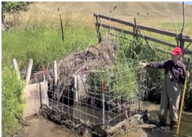
Photo showing an exclusion fence built similar to a culvert fence to protect a water diversion headgate in Montana. Photo from Clark Fork Coalition presentation: Virtual Field Trip: Non-Lethal Beaver Conflict Resolution YouTube (2021).
