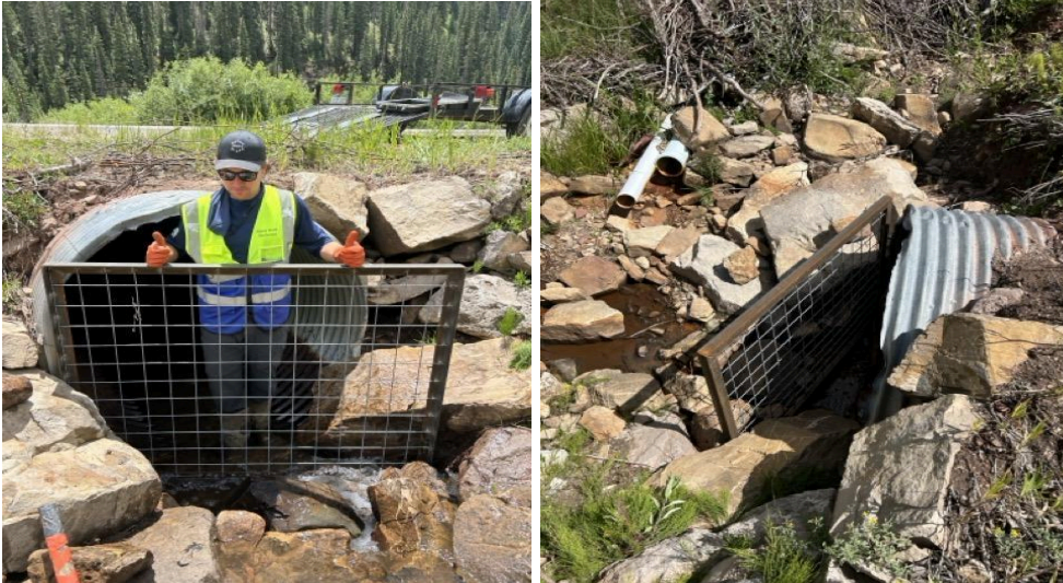
Photos by Rory Cowie, Alpine Water Resources, LLC, Silverton, CO, showing another example of how to allow for wildlife passage by off-setting the placement of a culvert protection panel.
