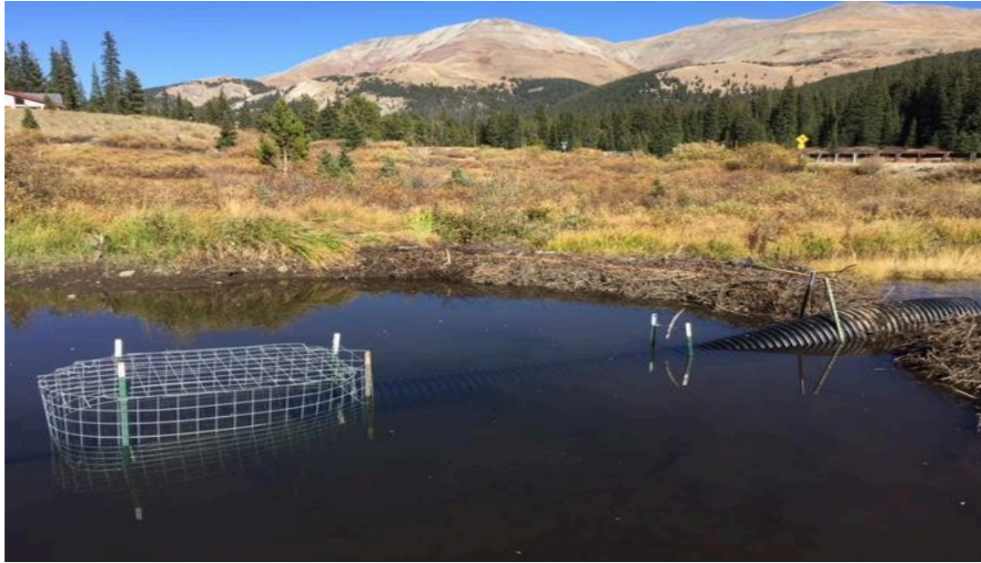
Figure 6-2. Photo of a flow pipe installed through a beaver dam by Summit County in 2018. The dam is located just upstream of Highway 9, at Summit County's Monte Cristo Open Space near Quandary Peak. Photo by Summit County Open Space and Trails staff. See Appendix B for more information and photos about this project.
