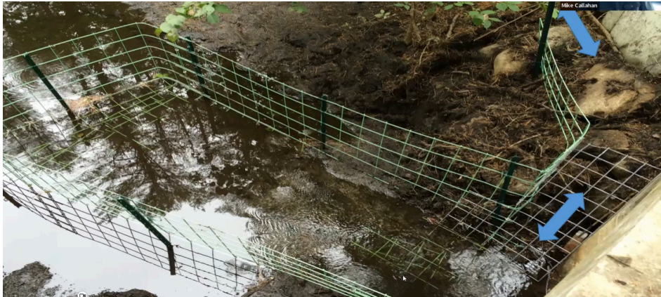
Photo from the Beaver Institute of a culvert exclusion fence that allows for wildlife passage as shown with the blue arrows.
