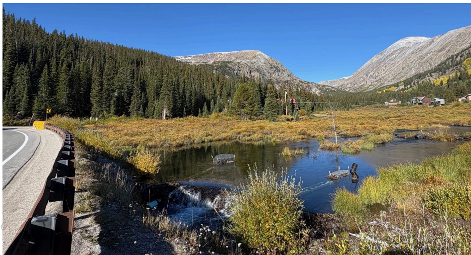
Photo of the same double flow pipe and culvert exclusion fencing taken in September 2025 showing beaver wetlands located adjacent to Highway 9. Photo by Summit
