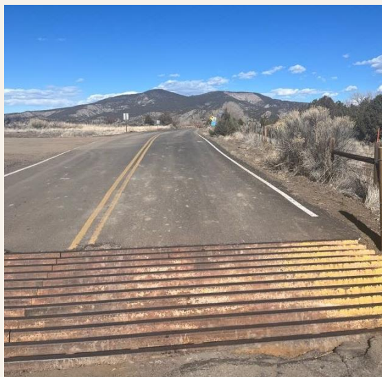
Figure 47. Recently paved CR 982 at the main entrance to Navajo State Park.
