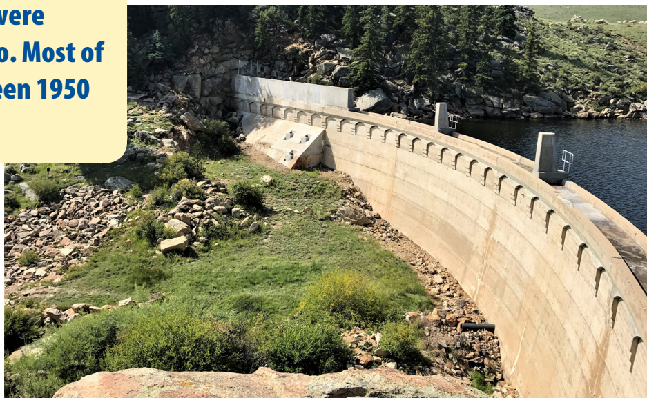
Tarryall Dam, Park County
