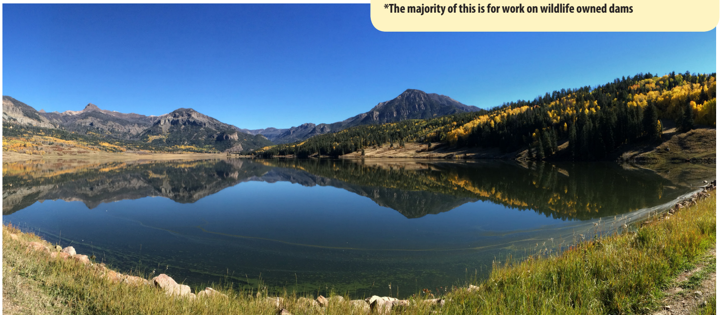
Williams Creek Dam, Hinsdale County
