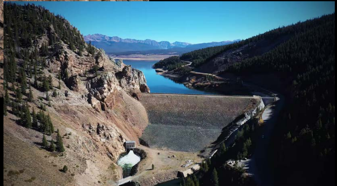
Uncompahgre Project - Taylor Park Reservoir
