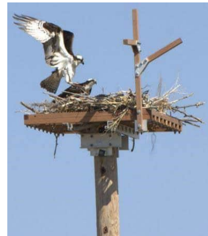
Figure 4-6. Raptor Nesting Platform in Laporte, Colorado
