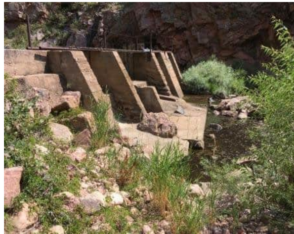
Figure 5-1. North Poudre Canal Diversion Structure
