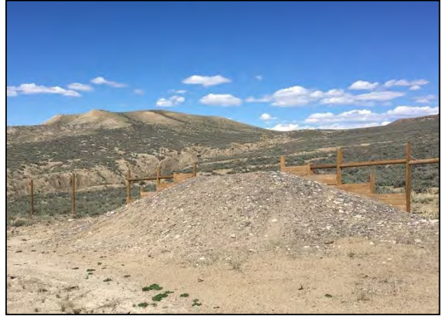
Figure 2-2. Example of an escape ramp with a 2:1 slope with perpendicular rail fence (left) and a ramp with a 3:1 slope without rail fence (right).
