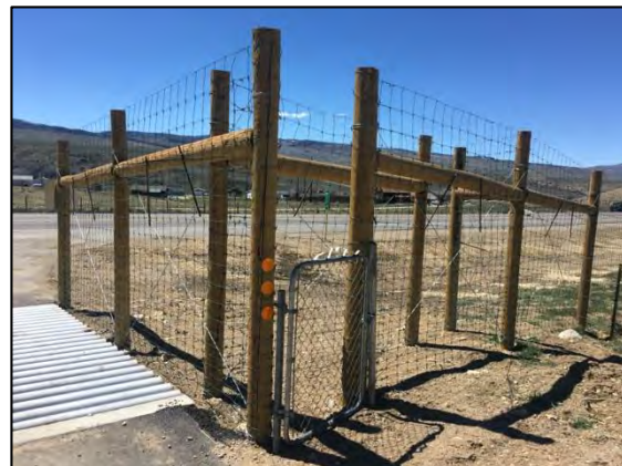
Figure 7-4. Pedestrian access point outfitted with a swing gate.
