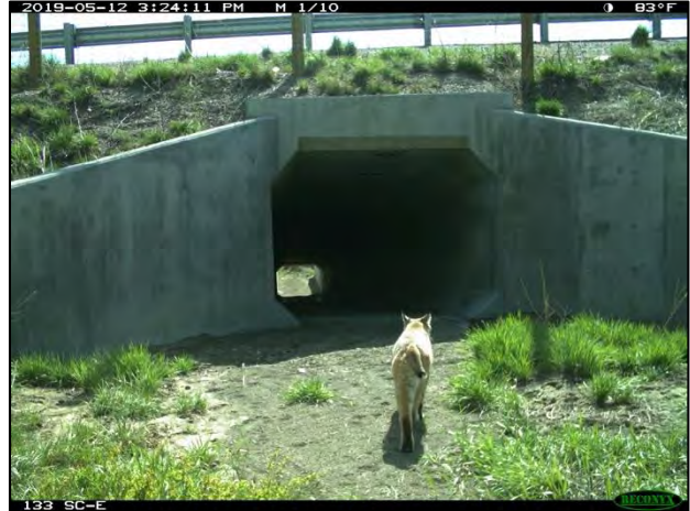
Figure 4-16. Bobcat entering the BVR box culvert.
