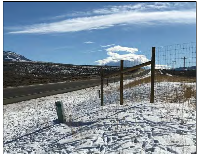
Figure 2-3. Cameras encased in utility boxes at the south fence end.
