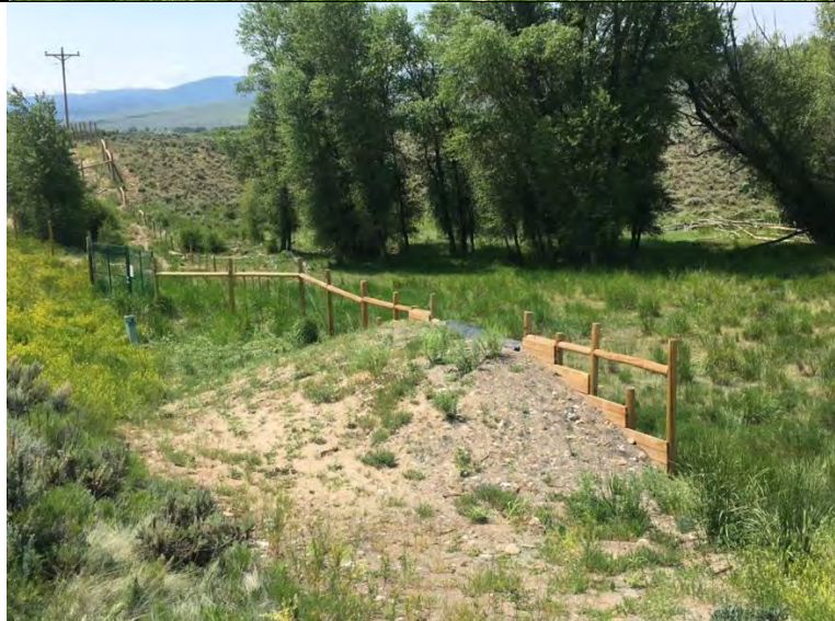
Escape Ramp – 3:1 slope without perpendicular rail fence
