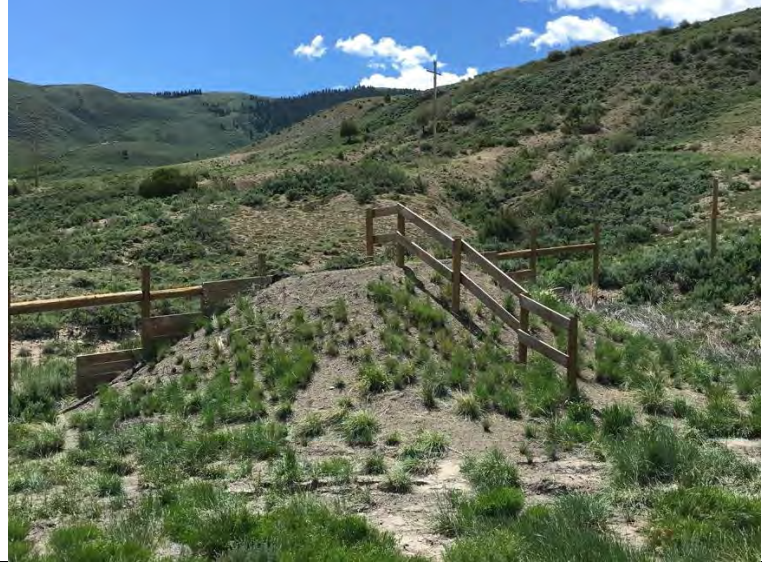
Escape Ramp – 2:1 slope with perpendicular rail fence
