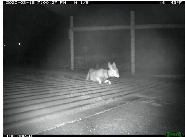
Figure 5-6. Mule deer that fell between the bars of a wildlife guard.
