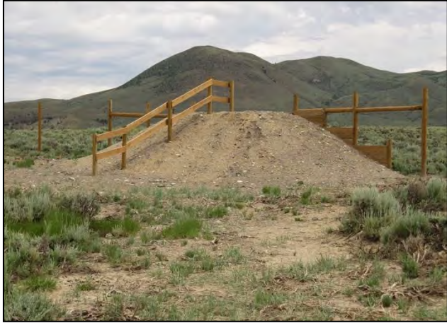
Figure 2-2. Example of an escape ramp with a 2:1 slope with perpendicular rail fence (left) and a ramp with a 3:1 slope without rail fence (right).
