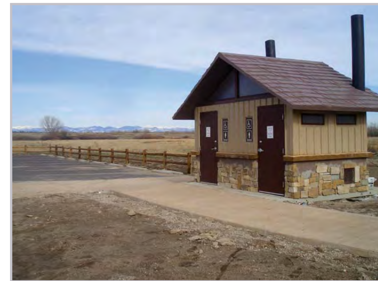
Improved restrooms and parking lots
