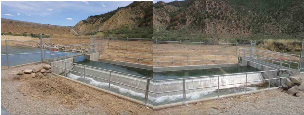
Figure 3. Rifle Creek fish screen. Structure is not "angled" as combined photographs suggest from side-view.
