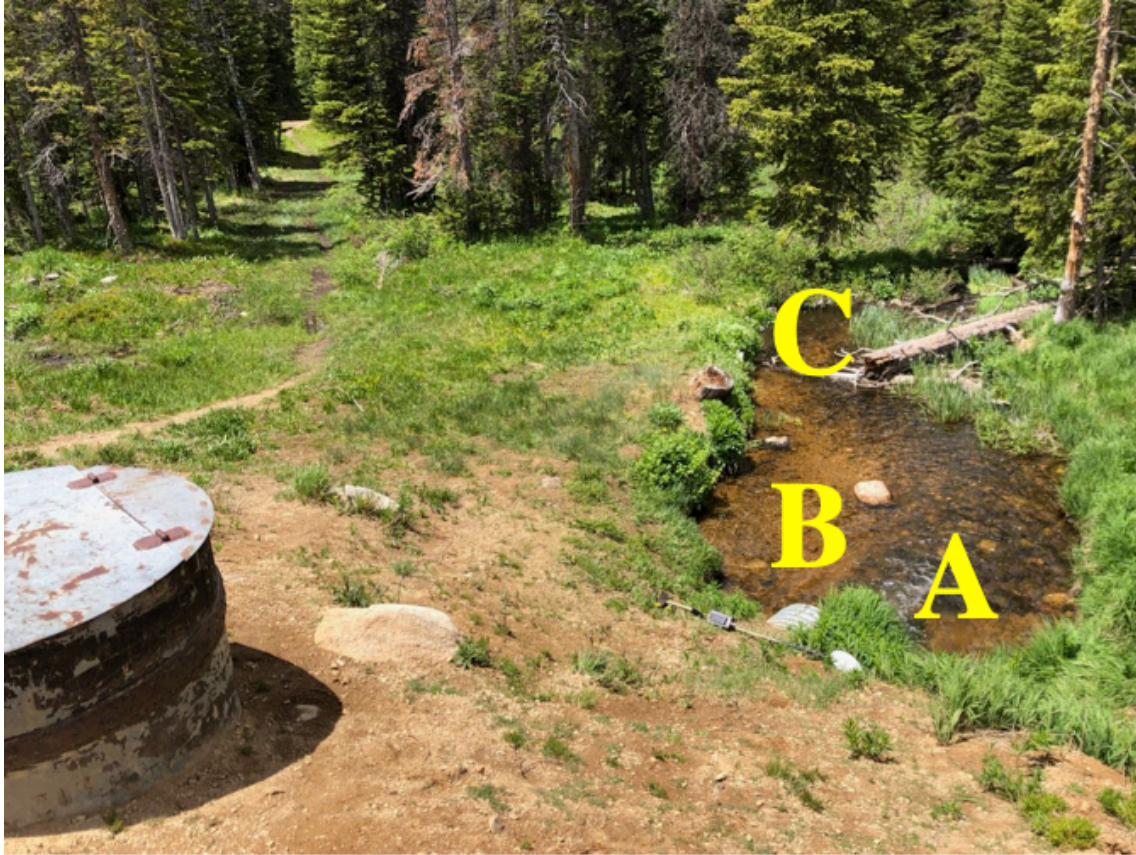
Figure 1. Antenna locations in the outlet pool below Zimmerman Lake. The outlet works are housed in the culvert in the bottom left of the photograph
