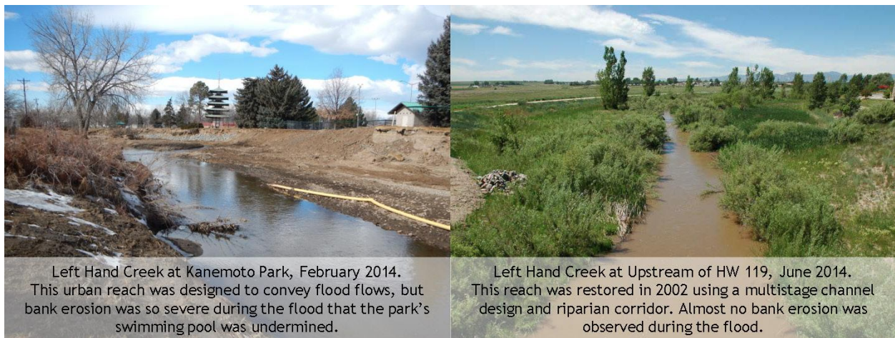
Figure 2. Pictures of the two locations on Left Hand Creek illustrating the value of multistage channel designs and functioning riparian corridors for flood conveyance and channel stability.
