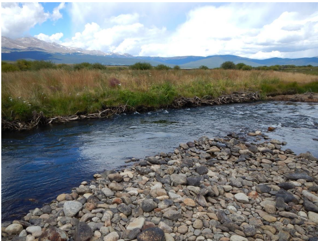
Figure 7.6. Typical wood-toe/sod mat structure used for habitat restoration on the Upper Arkansas River.
