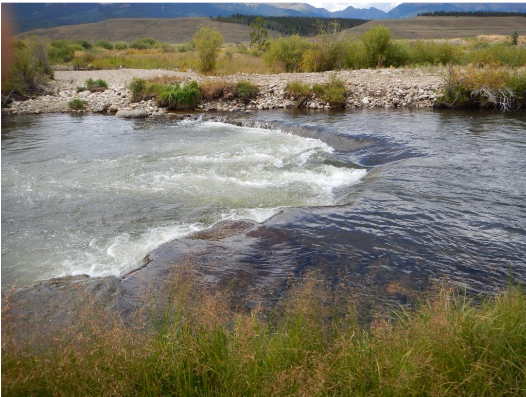
Figure 7.2. Typical cross-vane structure used during habitat restoration on the Upper Arkansas River.
