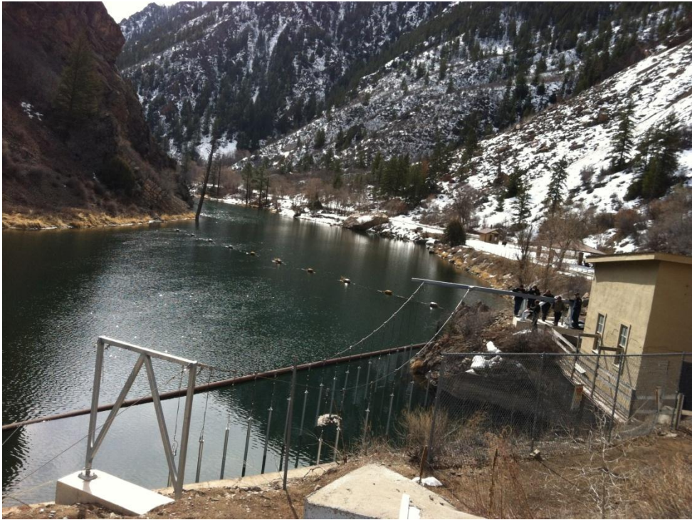
Figure 25. The electric fish guidance system on the east portal of the South Canal.
