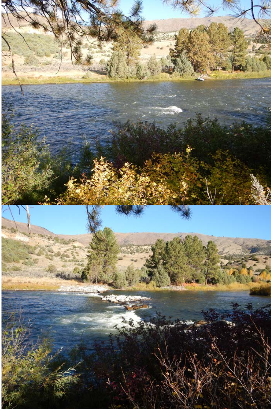
Figure 12. Before and after photos of the whitewater park feature at Pumphouse on the Colorado River. The whitewater park feature replaced a natural run with a drop structure featuring two hydraulic waves.
