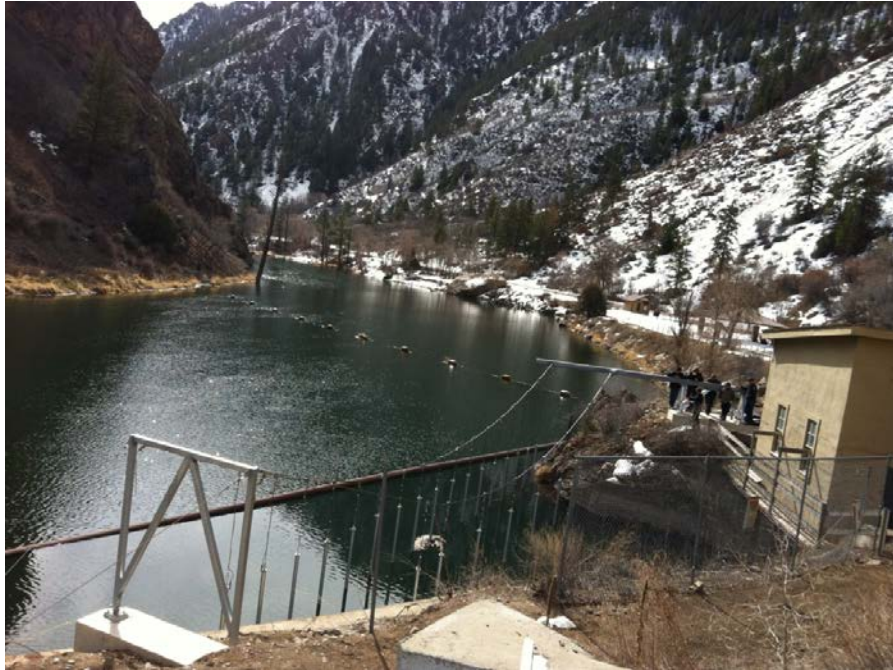
Figure 3. The electric fish barrier on the east portal of the South Canal.
