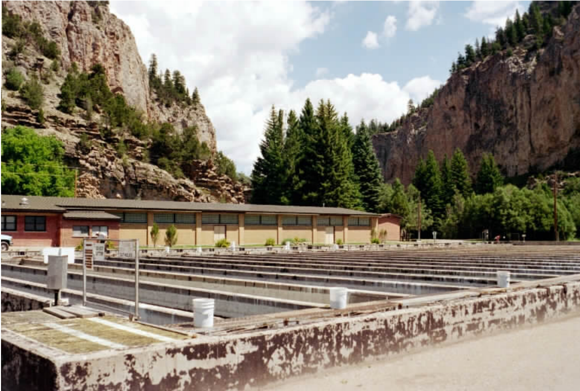
Figure A2.2. Rifle Falls Hatchery, with raceways and hatch-house pictured at left, is fed by a mix of 5 springs collected less than a mile from the hatchery. The right photo shows the area where the springs mix prior to entering the hatchery. The springs produce a consistent supply of water at a year-round temperature of 59°F.
