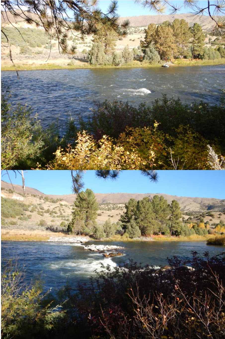
FIGURE 7. Before and after photos of the whitewater park feature at Pumphouse on the Colorado River. The whitewater park feature replaced a natural run with a drop structure featuring two hydraulic waves.
