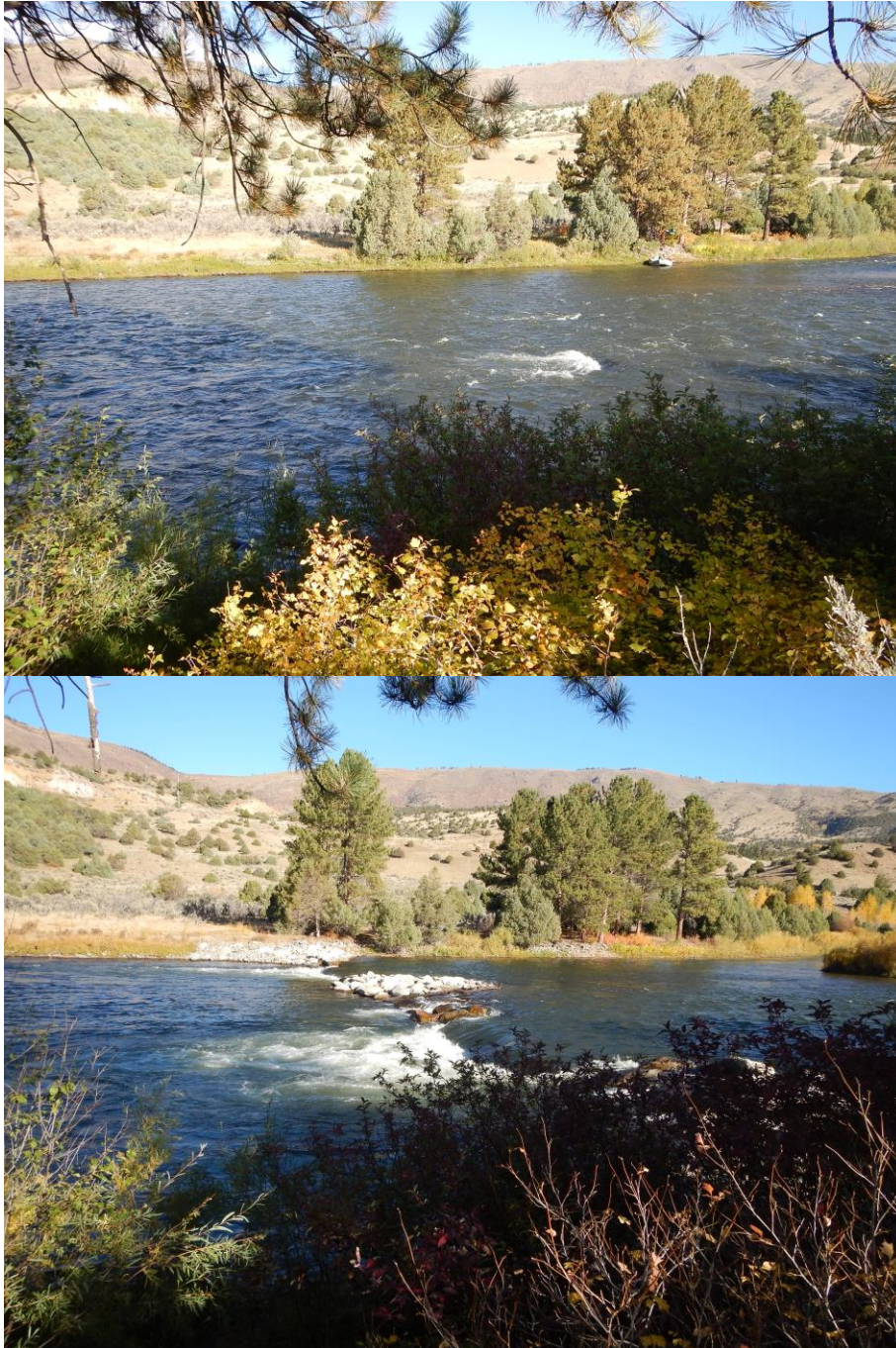
FIGURE 4. Before and after photos of the whitewater park feature at Pumphouse on the Colorado River. The whitewater park feature replaced a natural run with a drop structure featuring two hydraulic waves.
