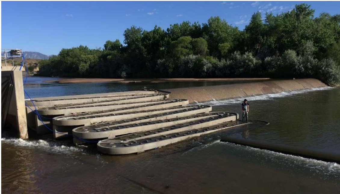
Figure 8. Fish passage structure on the Owens-Hall Diversion, Fountain Creek, Colorado. Note the technician at bottom of the passage structure for scale.
