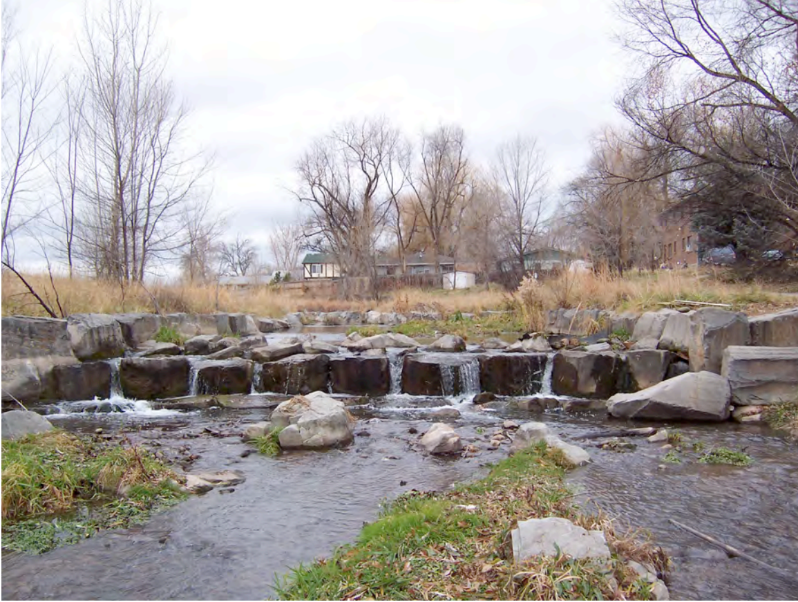
Figure 3.2 — The vertical drop structure on Spring Creek. This structure has an average drop height of 63 cm that prohibits non-jumping and small-bodied jumping fishes from moving upstream. Photo: Ashley Ficke
