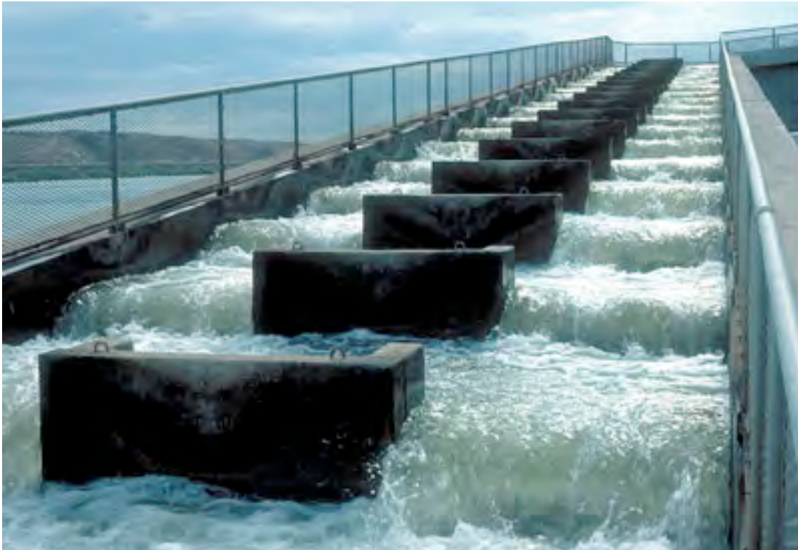
Figure 1.3 — Pool-and-weir fishway on the John Day Dam, Columbia River, USA. Fish using this structure must ascend it by jumping over each weir into the next pool. Photo: U. S. Department of Energy ( www.energy.gov ).
