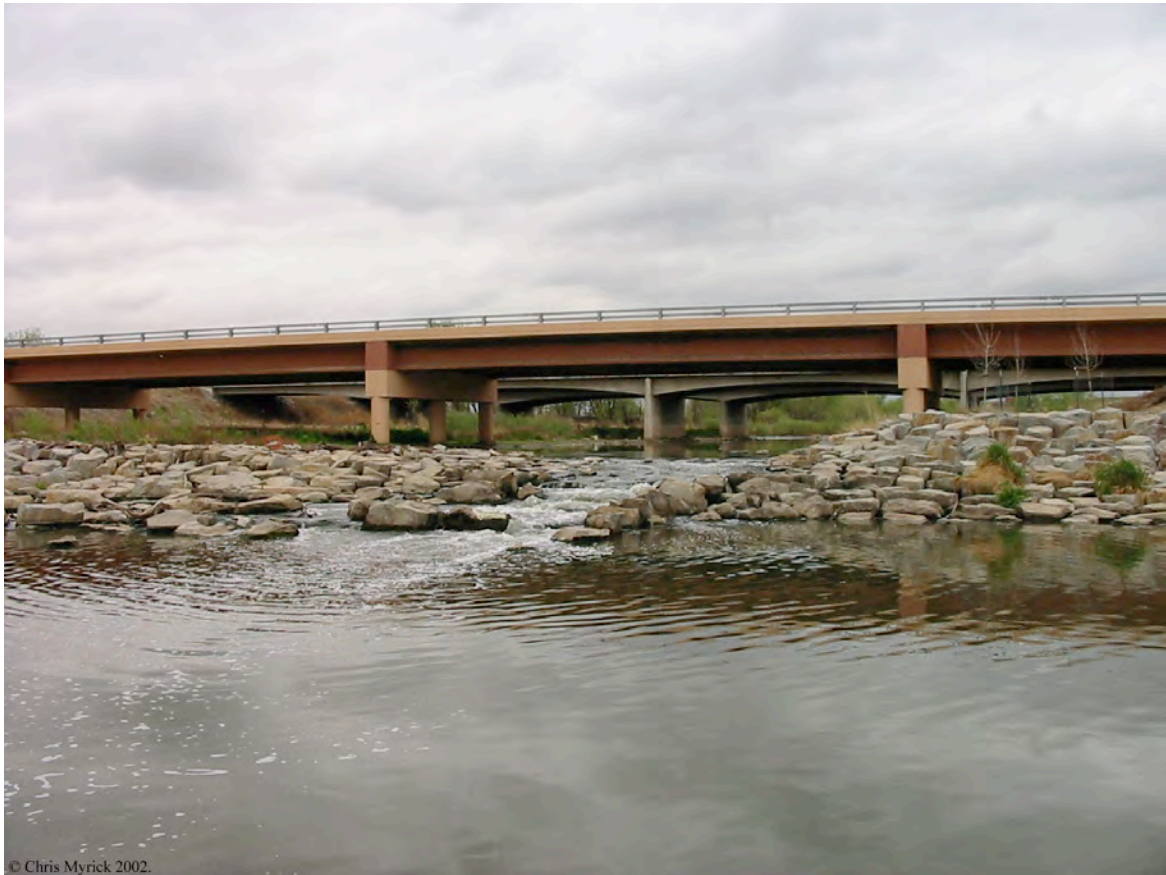
Figure 3.1 — A rock ramp fishway on the St. Vrain River, Colorado, USA. These structures incorporate a number of depths and water velocities, and they allow migration of non-jumping fishes. Photo: Christopher Myrick.
