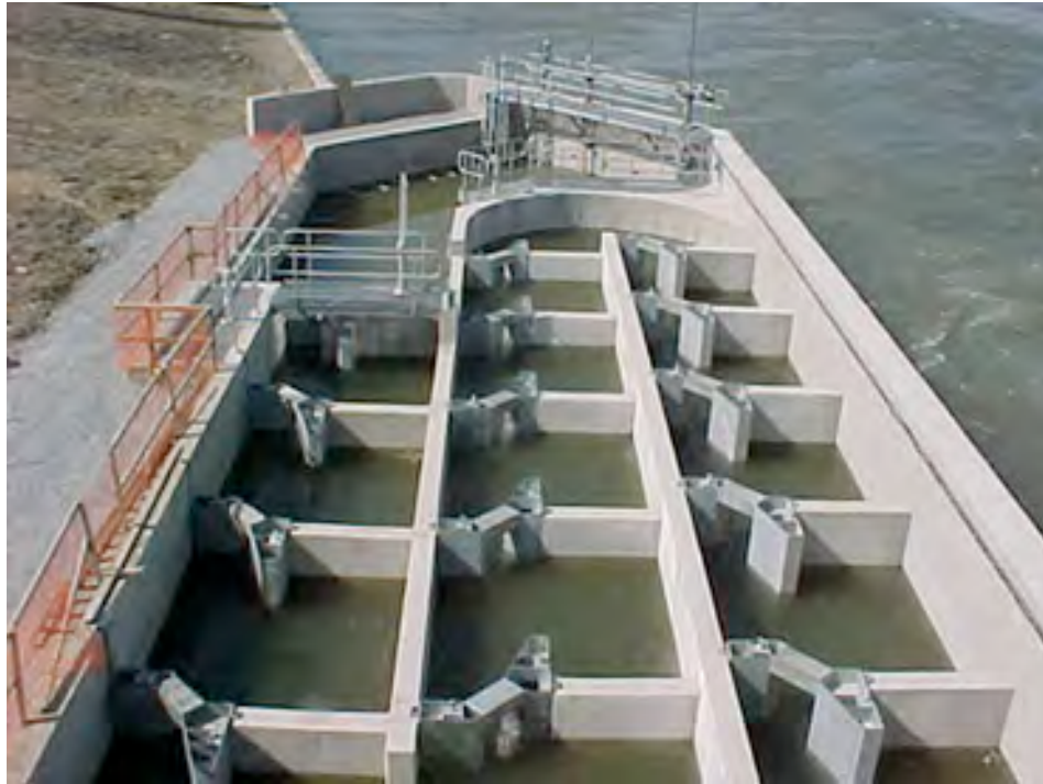
Figure 1.4 — Vertical slot fishway on the St. Ours River, Quebec, Canada. This type of structure does not require jumping, but water velocities in the vertical slot sections can be high. Photo: Parcs Canada ( www.pc.gc.ca ).
