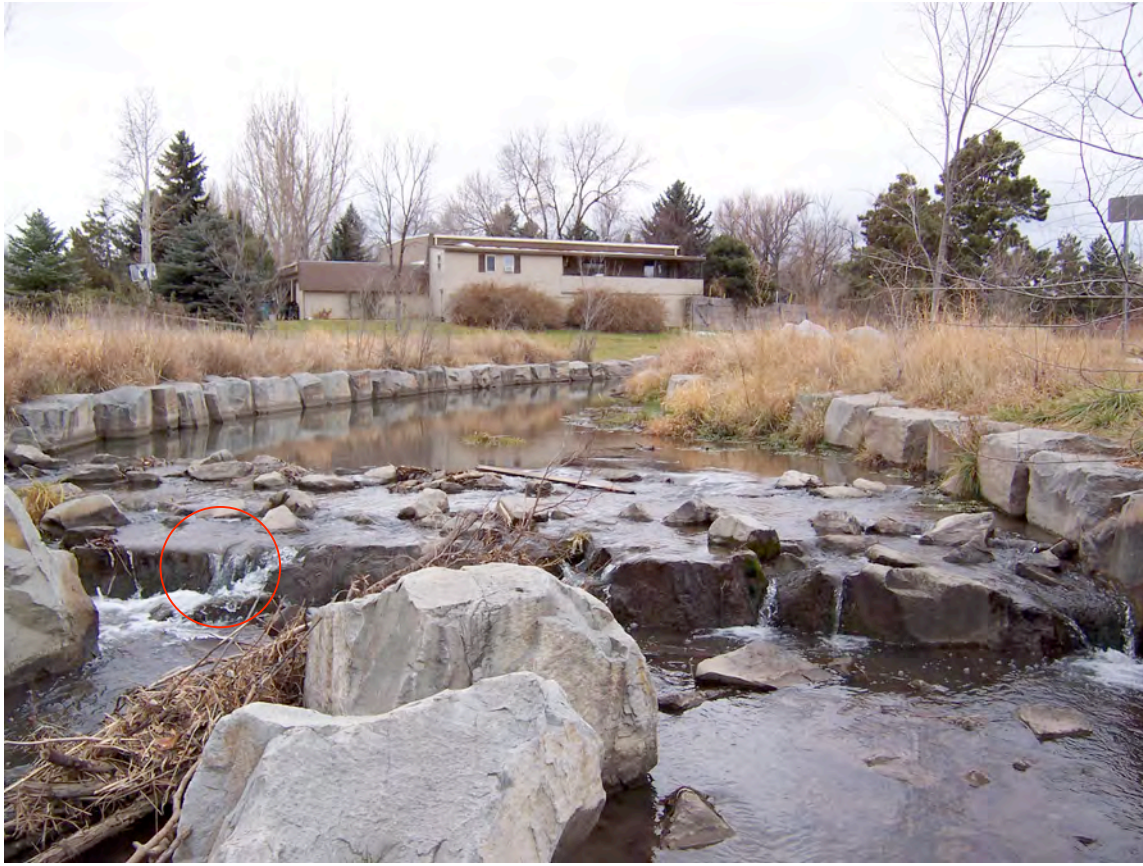
Figure 3.9 — The small cascade on Spring Creek. This structure incorporates a section (circled in red) that can be ascended by non-jumping fishes.
