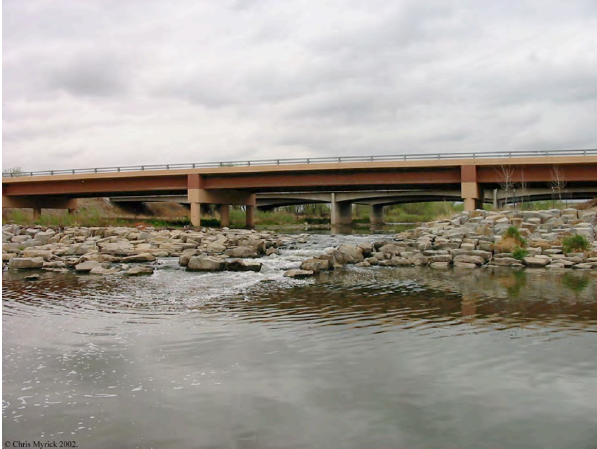
Figure 1.6 —A rock ramp fishway on the St. Vrain River, Colorado, USA. These structures incorporate a number of depths and water velocities and allow the migration of non-jumping fishes. Photo: Chris Myrick.
