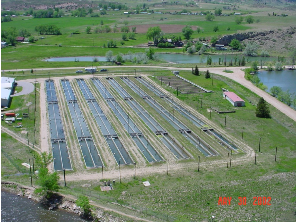
Figure A4.1. Watson hatchery uses surface water from the Cache la Poudre River, visible in bottom left corner. The water is diverted into a Watson Lake (visible to the right of the road on right side of picture) before coming into the raceways. We sampled fish from Watson that had previously resided at Bellevue, less than a mile away. Photo provided by Jim McKissick, CDOW.
