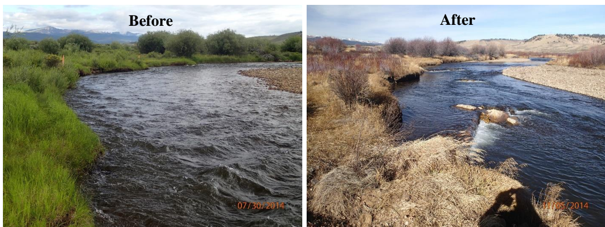
Figure 3. Before and after photos showing log vanes, habitat boulders, and channel narrowing.
