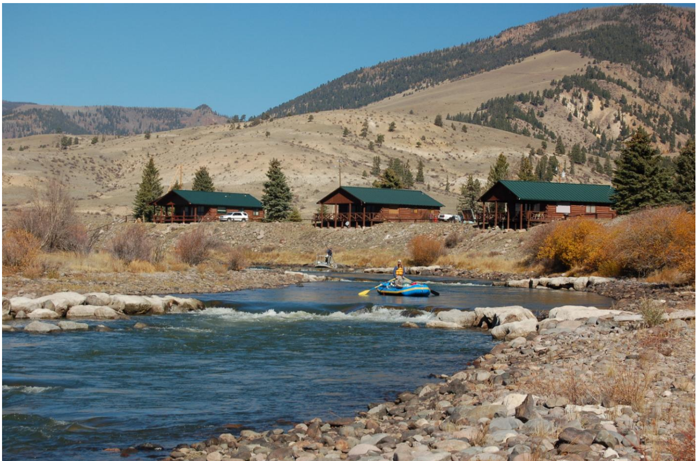
Figure 1. Upper Wason: Representative photo of the Upper Reach of the Wason Ranch. Notice the periodic large boulder-constructed cross-channel structures (cross vanes) used for grade control, creating deep pools, and narrowing the channels.
