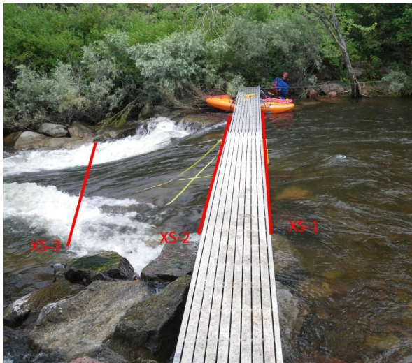
Figure 7: A. Velocity distribution profile through a typical WWP structure from St. Vrain Creek, Lyons, CO. Velocities were recorded using a flow meter corresponding to a discharge rate of 240 cfs. B. Locations where each of three cross-section velocity profiles were measured.
