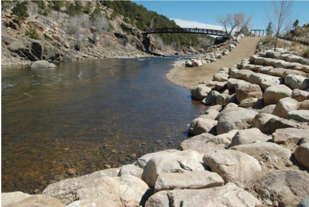
Figure 6. Typical lateral bank boulder armoring associated with WWP structures near Buena Vista, CO.
