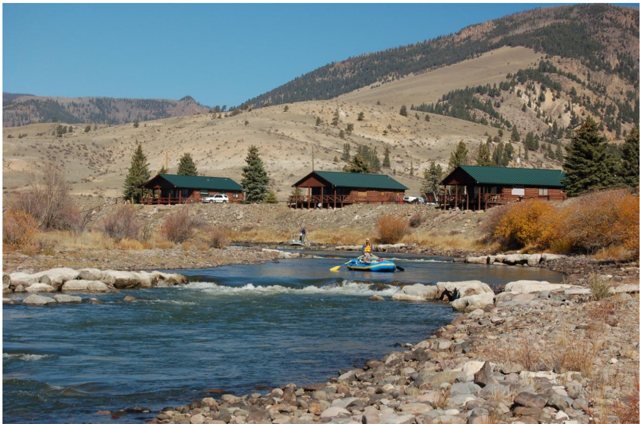
Figure 1. Upper Wason: Representative photo of the Upper Reach of the Wason Ranch. Notice the periodic large boulder-constructed cross-channel structures (cross vanes) used for grade control, creating deep pools, and narrowing the channels.
