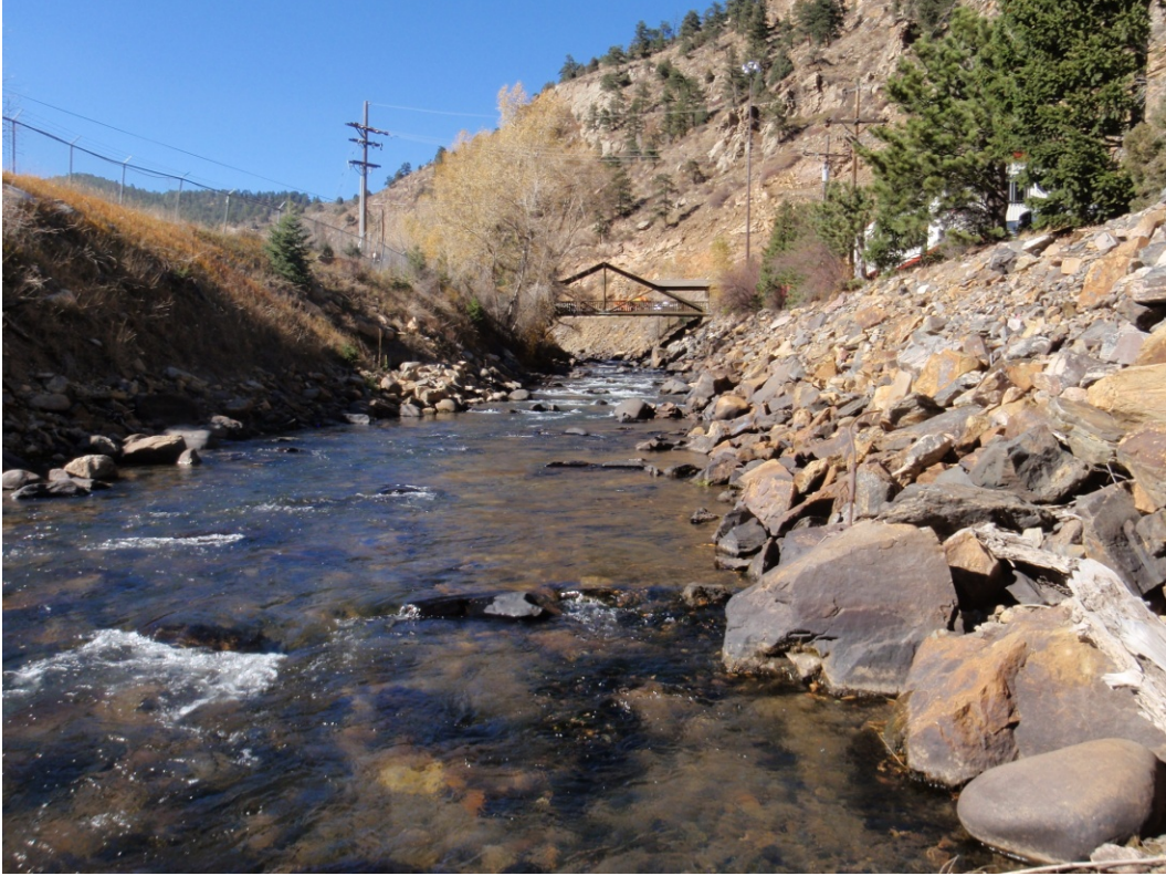
Figure 4. Example of trapezoidal channel that lacks riparian connectivity along Clear Creek.
