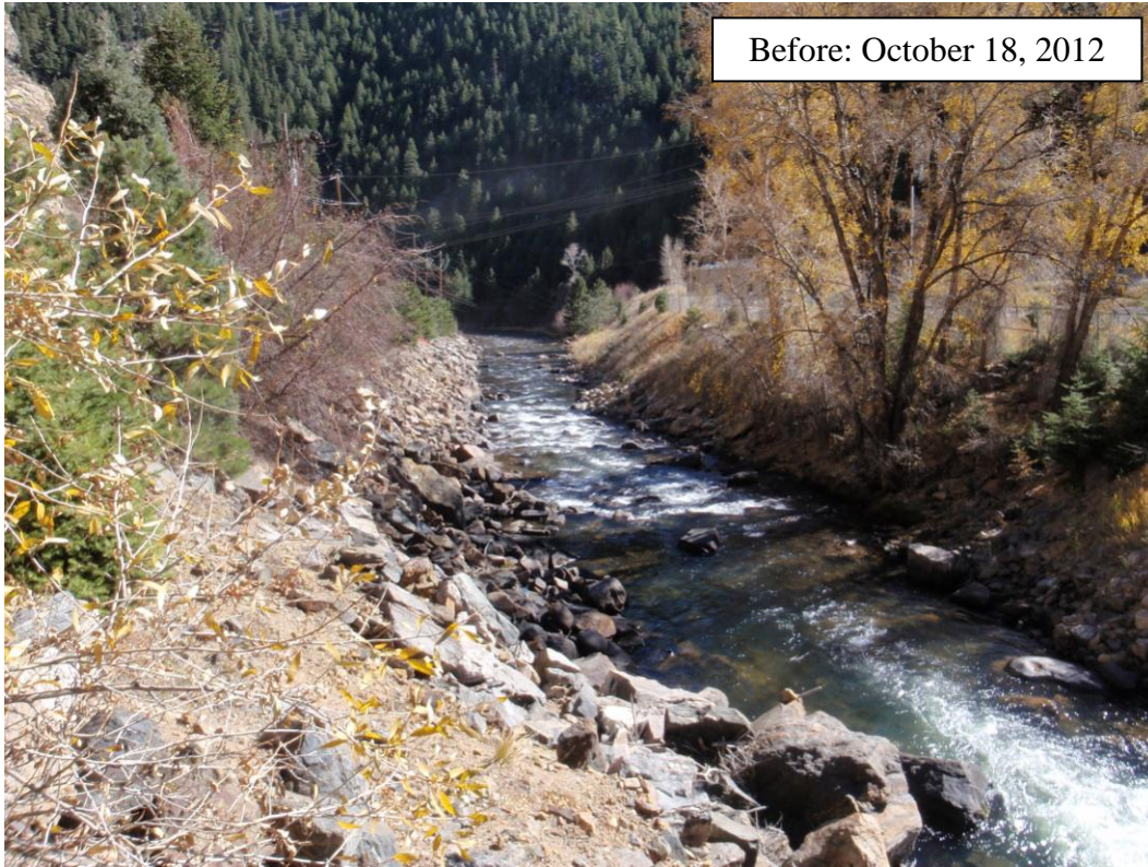
Figure 1.6. Pre-construction photo of the Twin Tunnels project site on Clear Creek.
