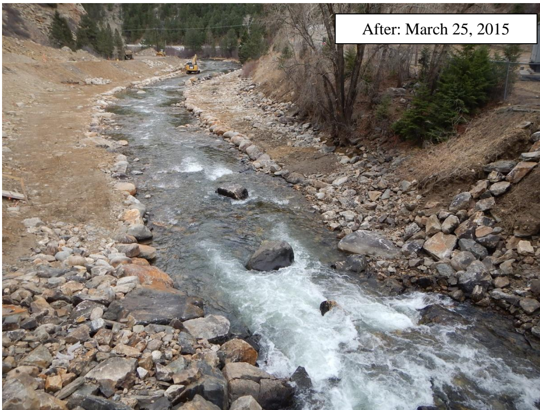
Figure 1.7. Post-construction photo of the Twin Tunnels project site on Clear Creek.
