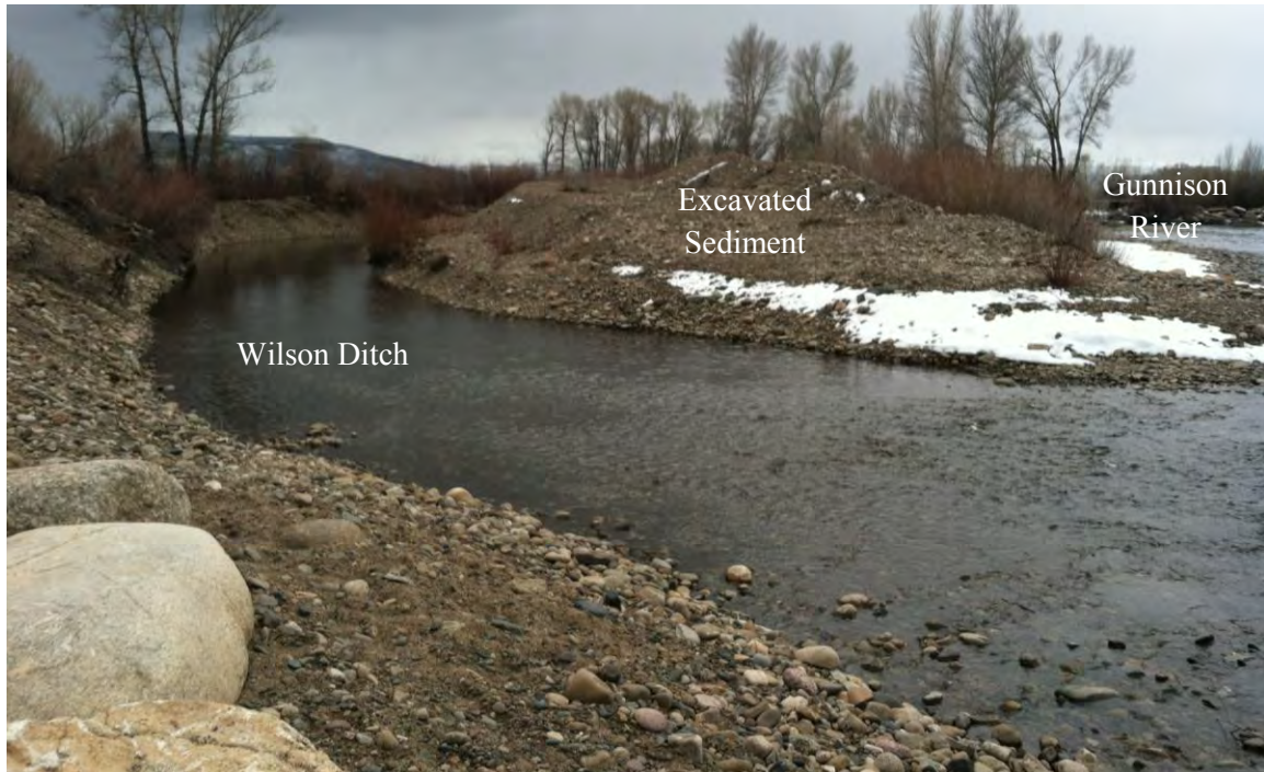
Figure 3. Inlet to the Wilson Ditch showing large pile of sediment that has been removed from the ditch and placed between the ditch and the Gunnison River.
